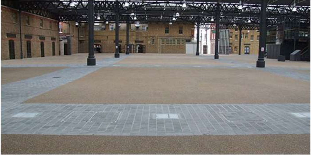
Addagrip Addaset Resin Bound Surfacing at Spitalfields Market, London – Brown colour tying in with natural stone blocks
